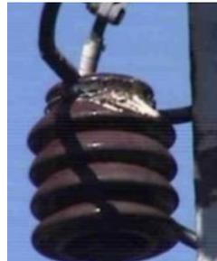
*Fig. 9, 10. Corona discharge and its effects.*
